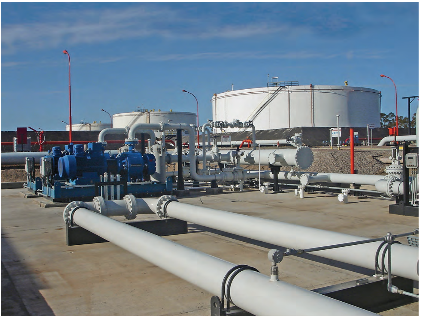
Onshore Terminal in Argentina
