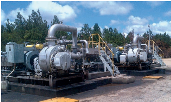
Multiphase Boosting System in high sand loaded Multiphase application
